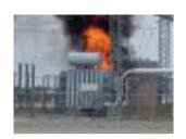
Transformer fires are a cause of concern and liability for electric utilities. An explosion usually takes place before fire. This results in loss of life and damage to the neighbouring equipments apart from causing power outage.
